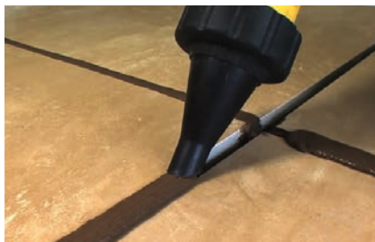
Grouting brick and tiles
