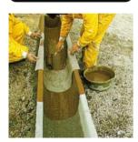
**Lastois canalones** is a product based on bicomponent resins and consistencies gel type, with great adhesion and elasticity ideal for the waterproofing of gutters.
