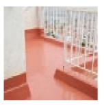
**Lastois MS Líquido** is a MS polymer-based waterproofing, which has very good waterproof properties on various support types and also on a wet surface. The product has a fast drying.
