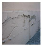
**Teais Capi C** is an injection system that is placed in the walls affected by moisture by capillarity. The system consists of making perforations with a drill in the wall or should be placed the injectors. The injected liquid has a high penetration and cures in a moist environment forming a barrier that prevents the access of the capillarity in the facing. The system allows repairs in the walls of stone, concrete, hollow and massive brick.
