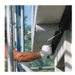
**Lastois capa intermedia** is a product based on elastomeric resins, additives and pigments with high resistance to water properties. It is easy to apply because is one-component. Efficient as a waterproofing.
