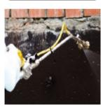
**Brepois** is a two-component epoxy tar that once is blended in proportion of 10 A / 1B on weight allows apply the product in thick coat avoiding dripping (150 microns per coat of wet film).
