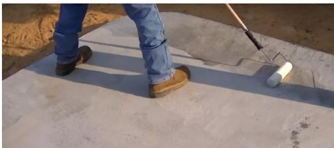
Application of IMPRIDUR on a screed with vapour barrier.
