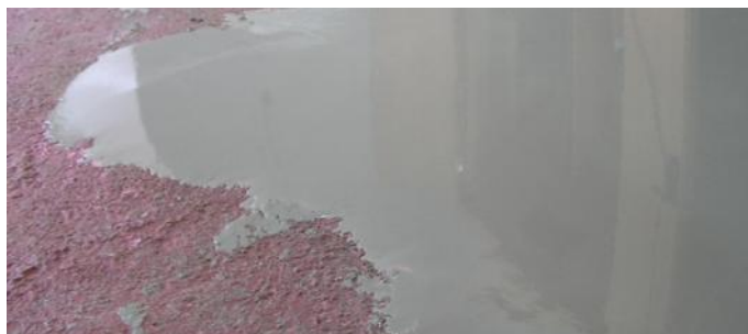
Application of DUREPOX self-levelling on screeds without vapour barrier.
